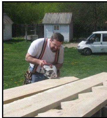
Steve Rutherford working on stairs
