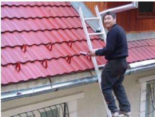
Ianco installing protective snow barriers.
